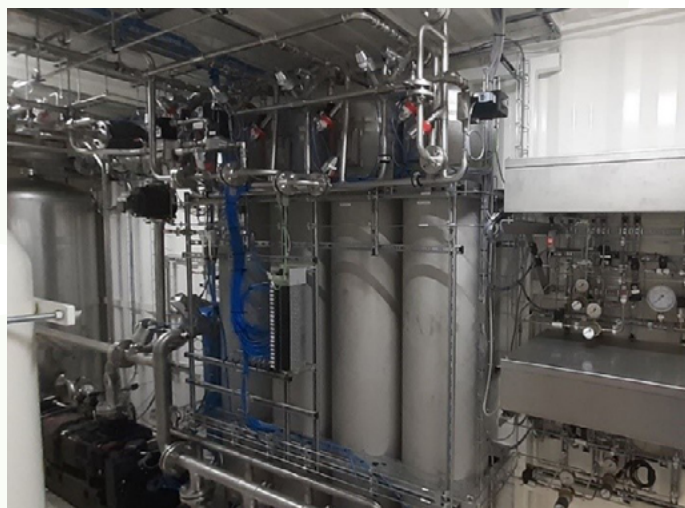
Installed To-Syn-Fuel PSA. Credit: Hygear.
